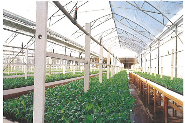
Greenhouses built by the Jain Group
